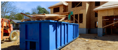
ROLL-OFF DUMPSTERS FOR: CONSTRUCTION DEBRIS
